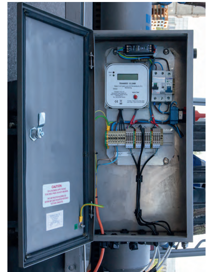
Figure 11. The Webserver Monitoring cabinet
